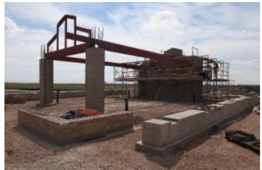
Rebuilding of the Committal Shelter
